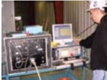
MV / LV cable insulation testing
